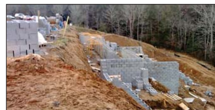
New Creekside Town Home popping out of the ground on Site 81
